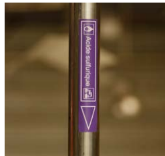
Pipes identification
