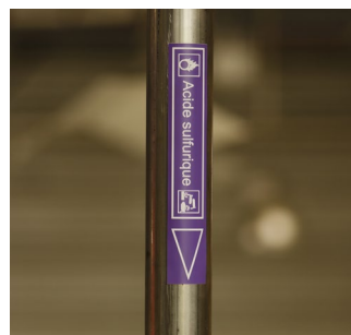
Pipes identification
